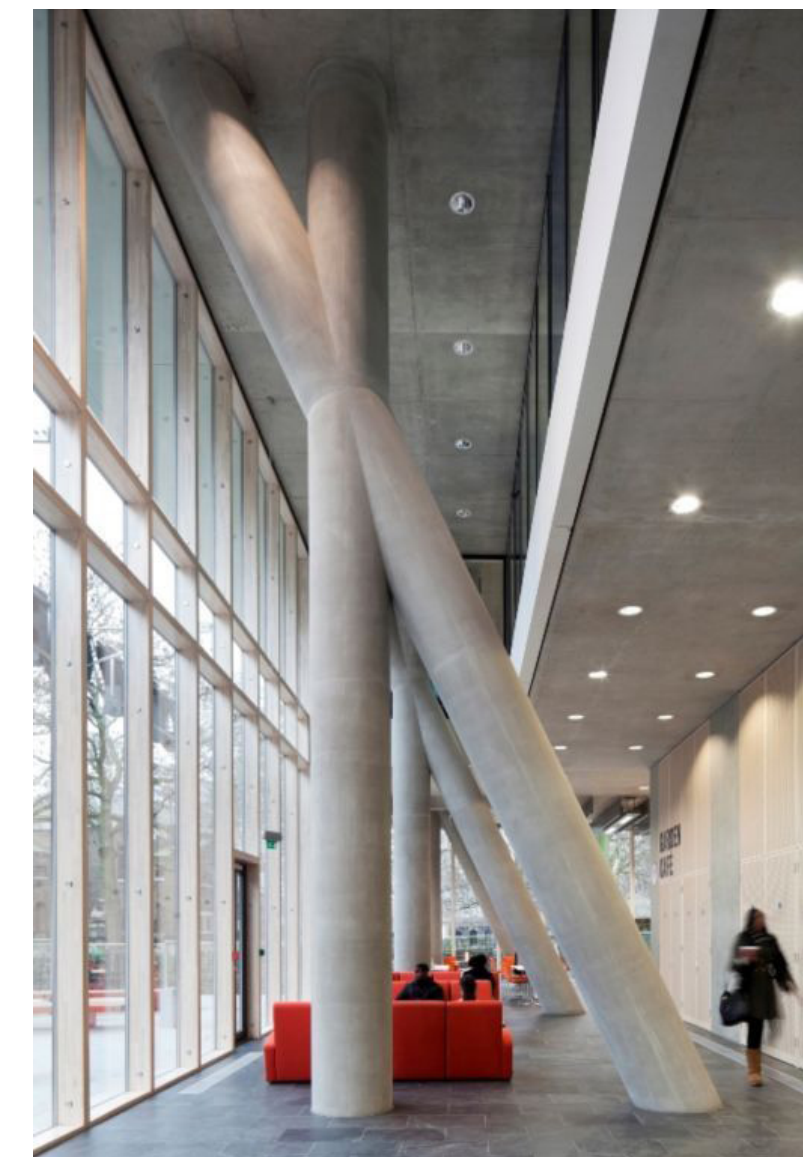
Concrete Column & Glass Window Wall
